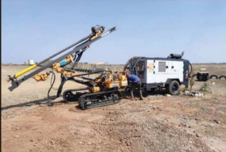
Blast Hole Drilling
